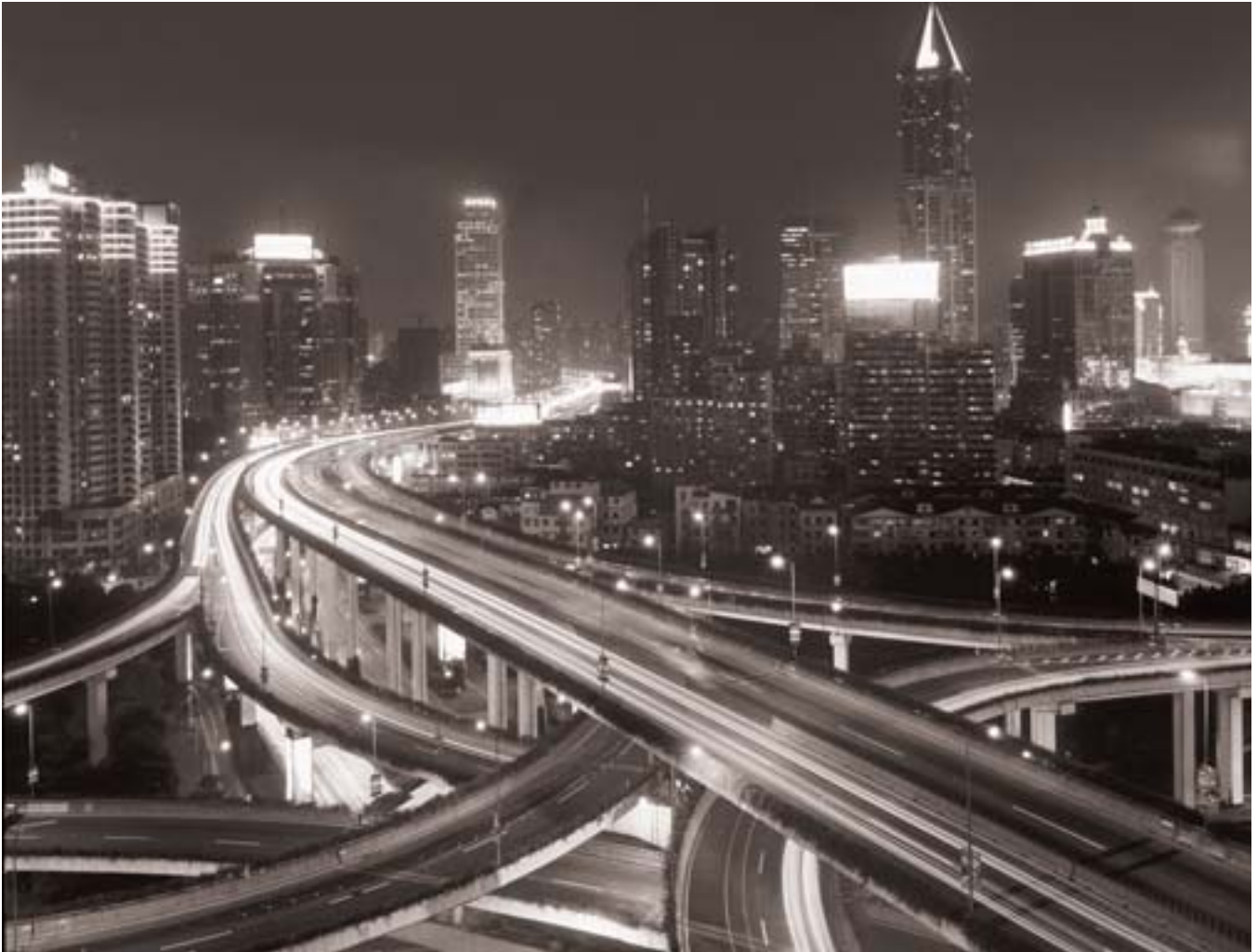
▲ Night view of urban highways and overpasses in Shanghai, China.
